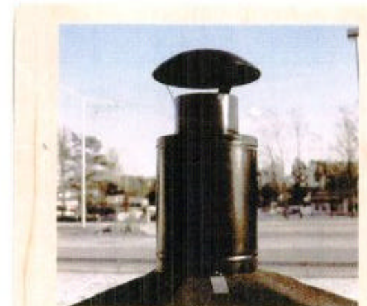
Chimney with waterproofing
